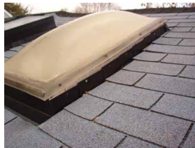
Incomplete flashing
