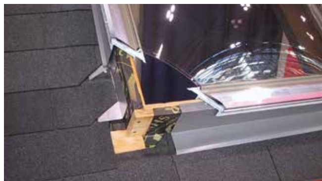
A curb mounted skylight
