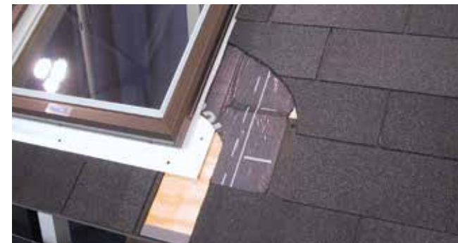
A integral-curb skylight installation
