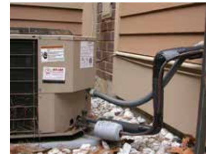
A typical filter/dryer - ensure that arrow is facing away from condenser
