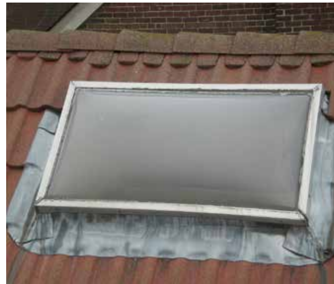
Skylight on tile roof
