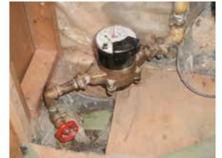
A jumper wire is needed here
