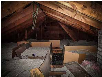
Photo: Attic insulation in older homes may contain asbestos that could fall through ceiling cracks. Courtesy Asbestorama
