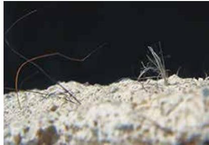
Photo: Drilling into drywall containing asbestos will release fibers into the air. Courtesy Asbestorama
