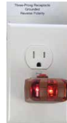
Grounded Circuit with Polarity Reversed
