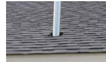
Missing Flashing
