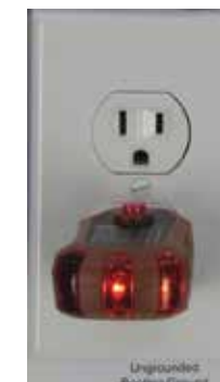
Left: 3-Prong with Bootleg Ground Tests as OK.
