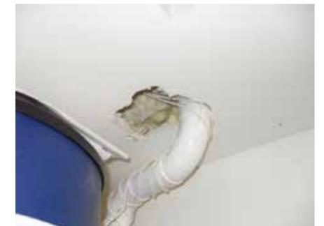
As you go into the garage, be clear as to exactly what parts of the garage connect to living space. Is it one wall, two walls, three walls? Is it all or part of the ceiling? Look for areas where the tightness of the wall may have been breached or where inappropriate materials have been used.
