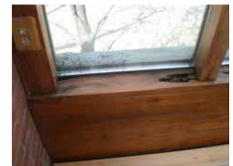
Water damage and rot on the interior sill of this window as a result of condensation – a common occurrence with single pane or poorly insulated glazing combined with high interior humidity levels.
