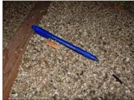
Vermiculite insulation commonly used in attics
