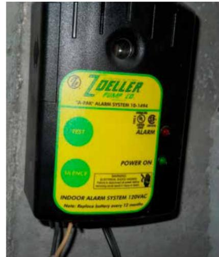
High water level alarm with battery backup. Connects to a float in the sump.
