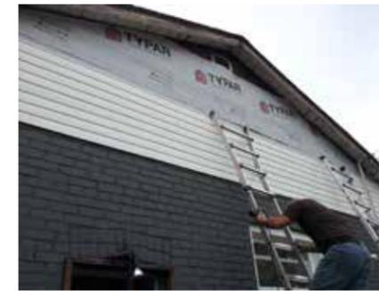
Although building paper can be used as an air, it is often ineffective because of loose joints
