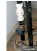
The other pipe is the pump discharge. Shortly after penetrating the cover there should be a check valve installed in the discharge pipe. Above the check valve should be a full-way shutoff valve (usually a ball or gate valve). This shutoff is required and is important to the person who is retained to replace the check valve and or disconnect piping to work on the pump.
