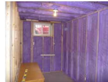
Foamed-in place insulation commonly used to increase R-value
