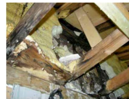
The water damage, mold and rot inside of this exterior wall assembly was a result of the extreme moisture from an indoor pool that was not properly managed – This structure had to be torn down.
