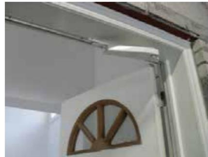
Here's a man door leading from the attached garage inside the house with an ineffective self-closer
