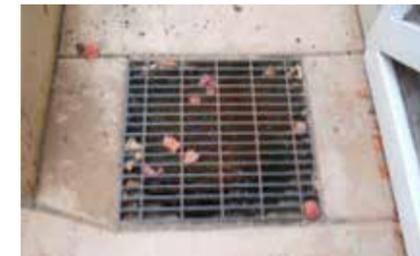
Exterior sump pump drainage grate cover
