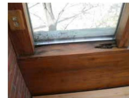
Water damage and rot on the interior sill of this window as a result of condensation – a common occurrence with single pane or poorly insulated glazing combined with high interior humidity levels.
