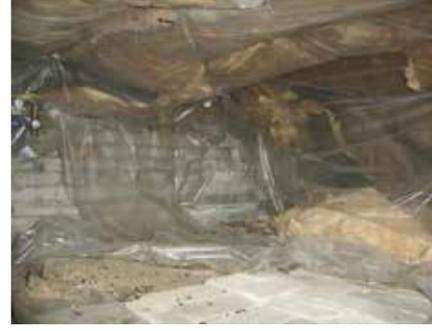
Here's a poorly installed vapor barrier on the ceiling of the crawlspace instead of the floor where it should be located.
