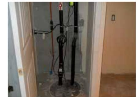
Sewage ejector in basement closet. Note check valve at discharge and shutoff
