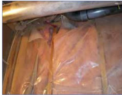
Damaged polyethylene film such as this is an ineffective vapor barrier, and an even more ineffective air barrier
