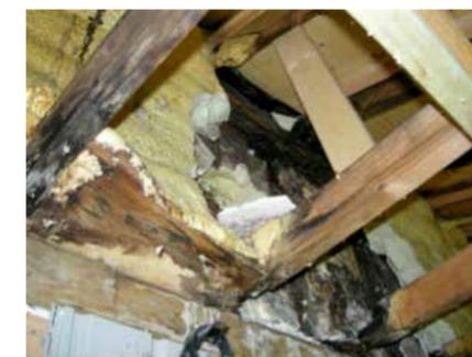
The water damage, mold and rot inside of this exterior wall assembly was a result of the extreme moisture from an indoor pool that was not properly managed – This structure had to be torn down.
