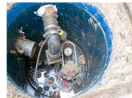
Sump pump at exterior, note high water level alarm float at discharge
