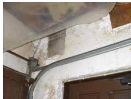
Here's some exposed foam insulation inside an attached garage that should be covered with drywall
