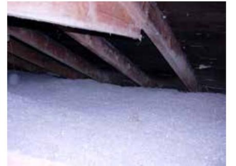
Blown-in cellulose also a common material
