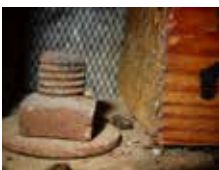
Circa 1950's Bolt – Some Powdery Surface Rust Only, 60 Plus Years Old and Performing Fine
