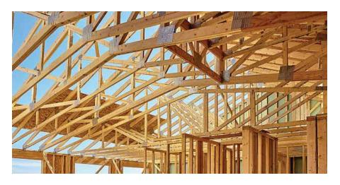
design. When components are left out or removed, the structural integrity of the truss and system is compromised.
