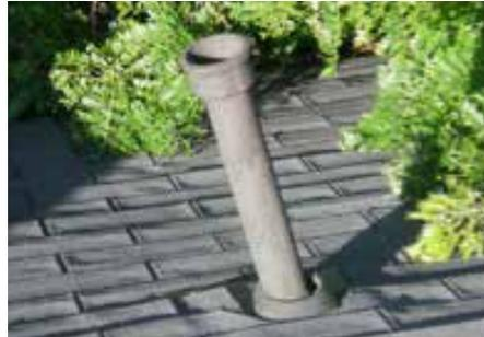
Improper support of this heavy cast iron stack has allowed it to drop. The flashing is not weather tight.
