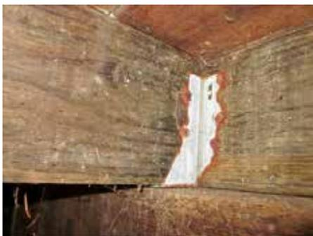
*Heavily Corroded Joist Hanger*
