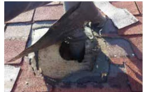
*Stack flashing and shingles damaged by vermin.*
