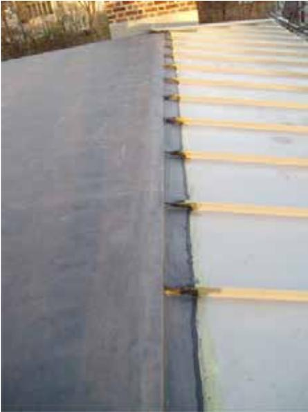
*Sloped standing seam metal roof connected to flat roof*
