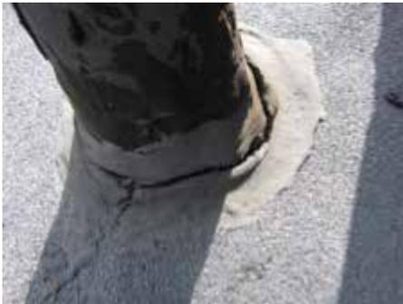
Roofing cement was used as the flashing material for this roof - a very poor approach, and over time has been damaged by UV exposure.
