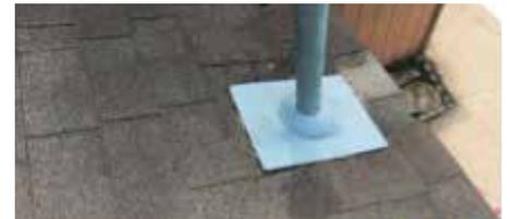
The entire flashing flange is on top of the shingles.
