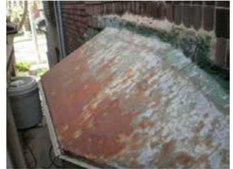
*Severely rusted sheet metal roof*
