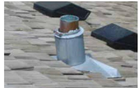
*Raccoons have chewed the lead collar. Tree branches should be cut back away from roof to help restrict raccoon access. The flashing sleeve and collar should be replaced.*
