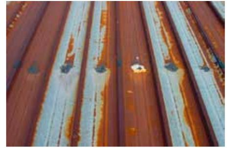
Rusted metal and failed fasteners
