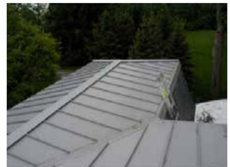
Standing seam low-slope metal roof
