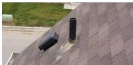
Buckling of the flashing can result in entry of vermin.
