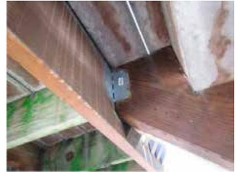
*Angle Clips Are Improper, There Is Some Separation Visible, Note Over Notched Tread Cuts*
