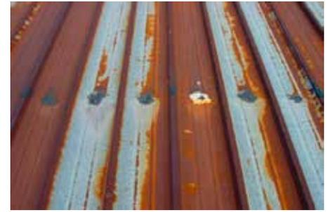
Rusted metal and failed fasteners
