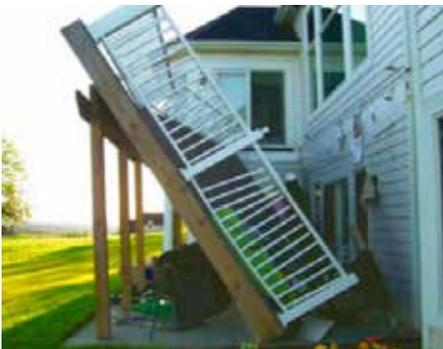
*Deck Failure at Ledger Connection – Picture from Net*
