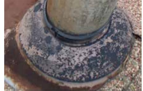
*This electrical mast flashing is rusted, and the rubber collar has failed.*
