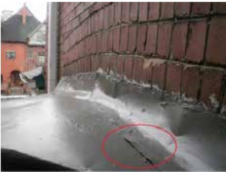
Open seams on this metal roof (poor roof-wall joint as well)
