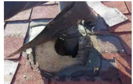
*Stack flashing and shingles damaged by vermin.*
