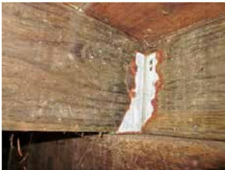
*Heavily Corroded Joist Hanger*
