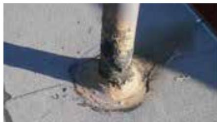
*This stack has rusted through, and roofing cement has been used to make a temporary repair.*
