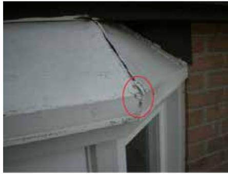
Open seams and rusted fasteners on this metal roof
