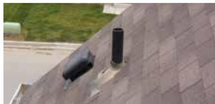
Buckling of the flashing can result in entry of vermin.
