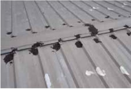
Caulking over leaking fasteners
