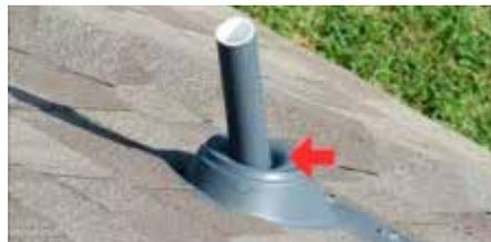
The flashing boot is recessed and will hold water.
