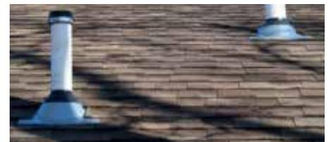
They forgot to remove the caps on the vents after pressure testing the drain system. A simple but urgent fix - remove the caps!
