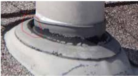
This is a common failure of the rubber collar. Collars often fail first on the uphill side of the vent.
