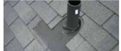
A poorly installed flashing may leak and will reduce its life expectancy.
