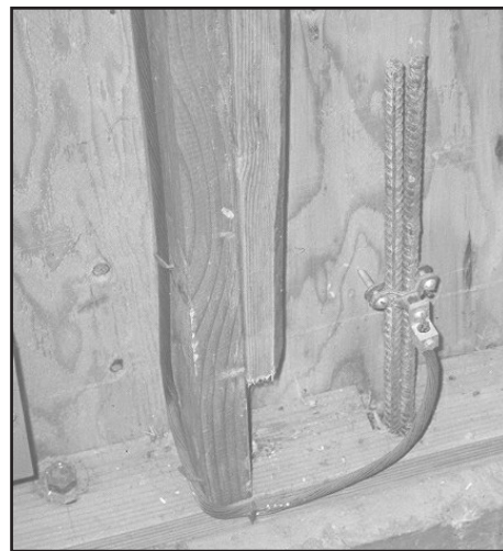
Figure 5 — Typical Ufer Ground
