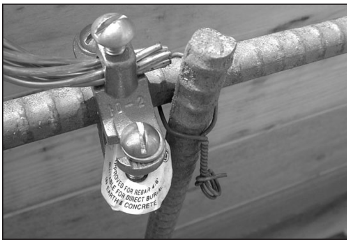
Figure 4 — Ground Clamp inside Foundation
